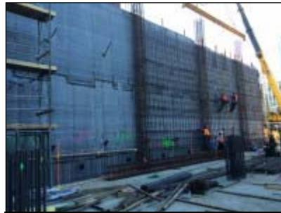
*Steel workers secure massive reinforcing cages into position at the first phase of the Metropolis project swings into high gear. AxisPointe is providing quality assurance services for the project.*
