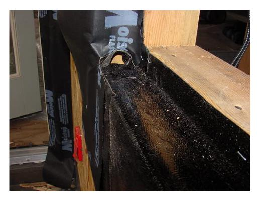
Splices lead to failure. Inside corners should be folded, not cut and spliced, to provide a leak-free joint. See sequence below.
