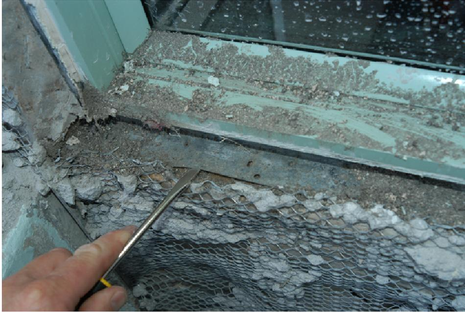
**This multi-million dollar window failure affected a seniors' care facility. Recessed window openings had reversed slope towards the interior, and missing waterproof components led to this failure.**
