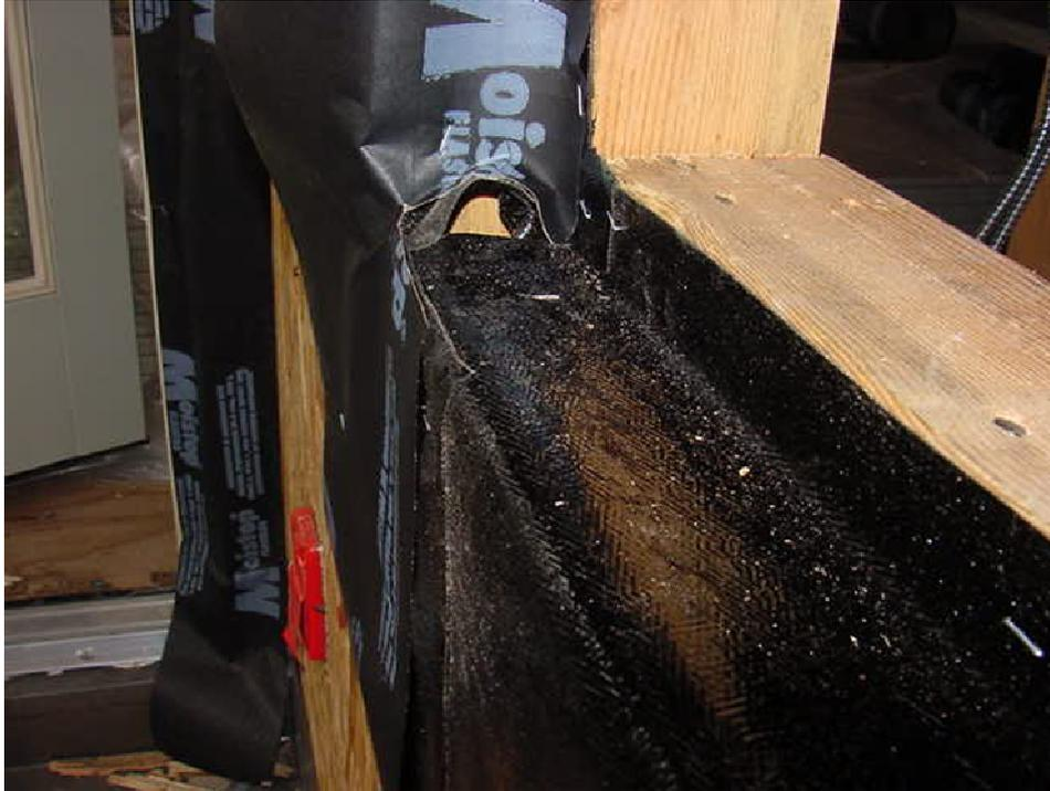
**Splices lead to failure. Inside corners should be folded, not cut and spliced, to provide a leak-free joint. See sequence below.**
