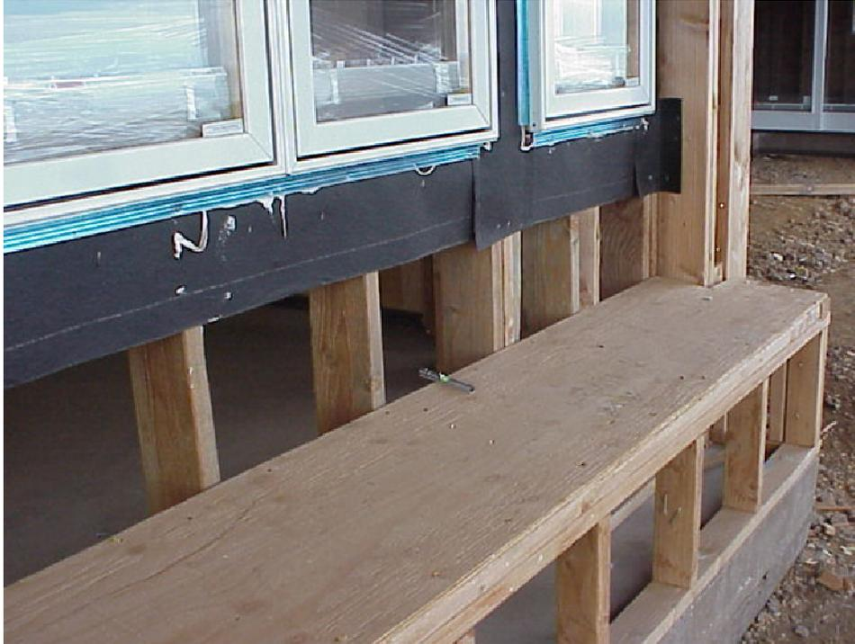
**Waterproof membranes require solid backing to provide support for the membrane.**
