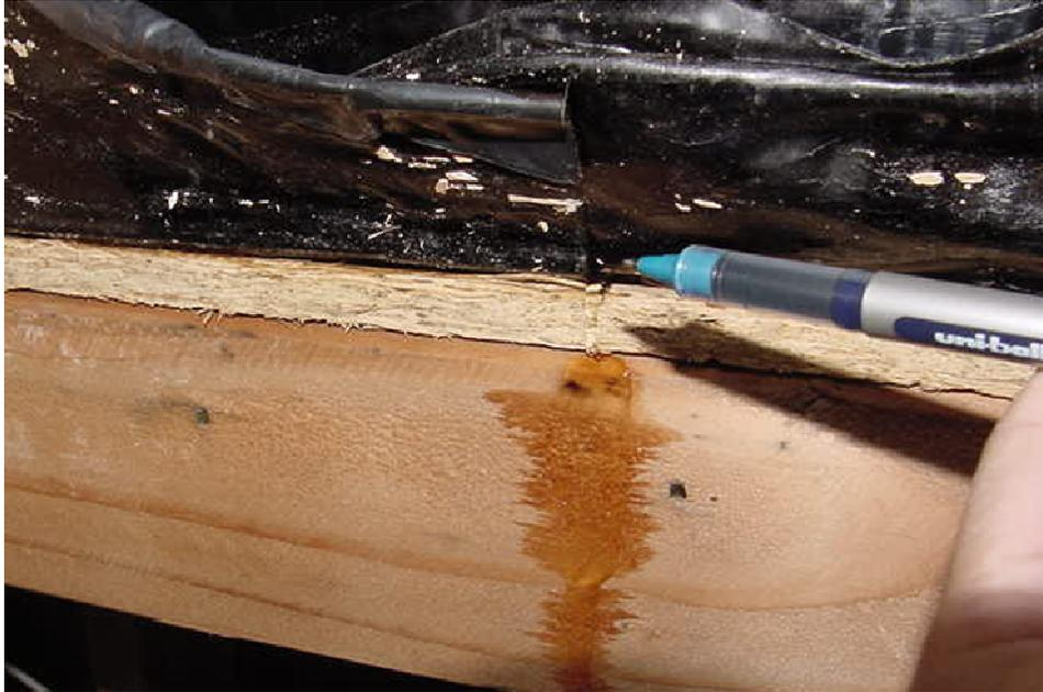
Inside the wall cavity, a flexible flashing membrane joint leaks into the building cavity. Inside 90-degree corners often leak here when the top membrane is not firmly pressed into the corner.
