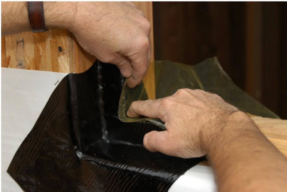
**Outside corners need additional waterproofing to eliminate a pinhole leak, installed prior to the SAF membrane. This non-reinforced SAF product contours to the complex corner, which will be covered with a reinforced SAF membrane.**
