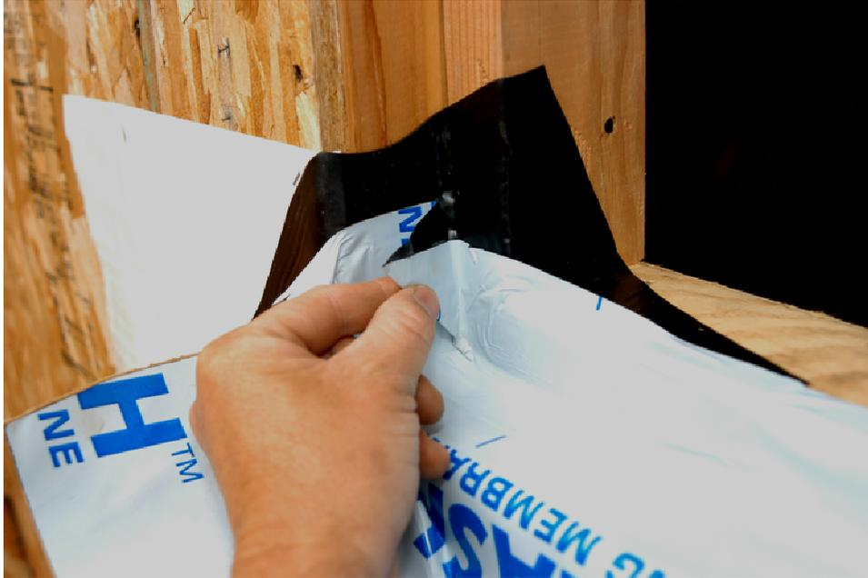
Inside corners can be folded instead of cut to eliminate leaks, as shown here. The next SAF membrane will cover the jamb and extend over this fold, creating a waterproof joint.
