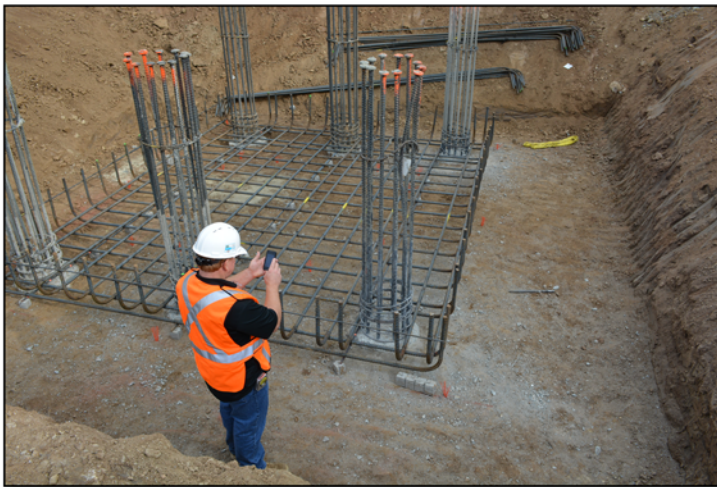
An AxisPointe employee inspects rebar footing, at the Metropolis job site in downtown Los Angeles, using an iPhone 4S with InSite Mobile
