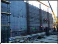
Steel workers secure massive reinforcing cages into position at the first phase of the Metropolis project swings into high gear. AxisPointe is providing quality assurance services for the project.
